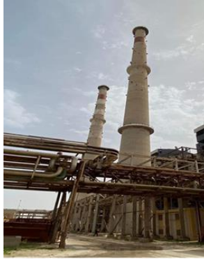
Figure 1. The Investigated Chimney at Tripoli-West Power Plant
